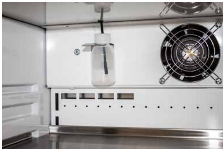
The P4 control sensor is installed in the bottle on the rear wall of the cabinet. Loosen the bottle cap to remove it from the rack.
